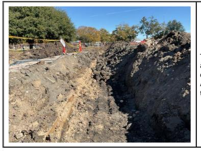
Top of soil to former asbestos piping containing cement. No Asbestos was present at time of inspection.
