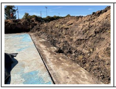
Top of soil to former asbestos cement sheeting. No Asbestos was present at time of inspection.
