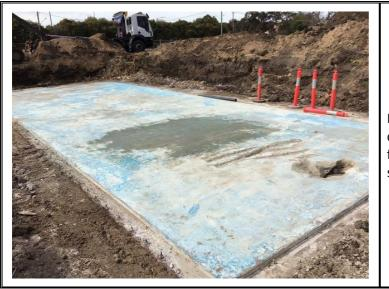
Northern Pool, top of concrete surface to former asbestos cement sheeting and debris
