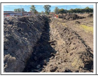
Top of soil to former asbestos piping containing cement. No Asbestos was present at time of inspection.
